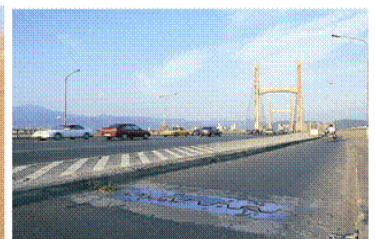
橋梁間的伸縮縫，使橋梁不致因熱膨脹擠壓而變形
